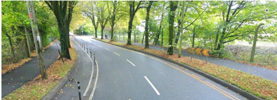
Figure 03.6 Images of Marquee Road (top) and Centre Park Road (bottom) (Google Earth)
